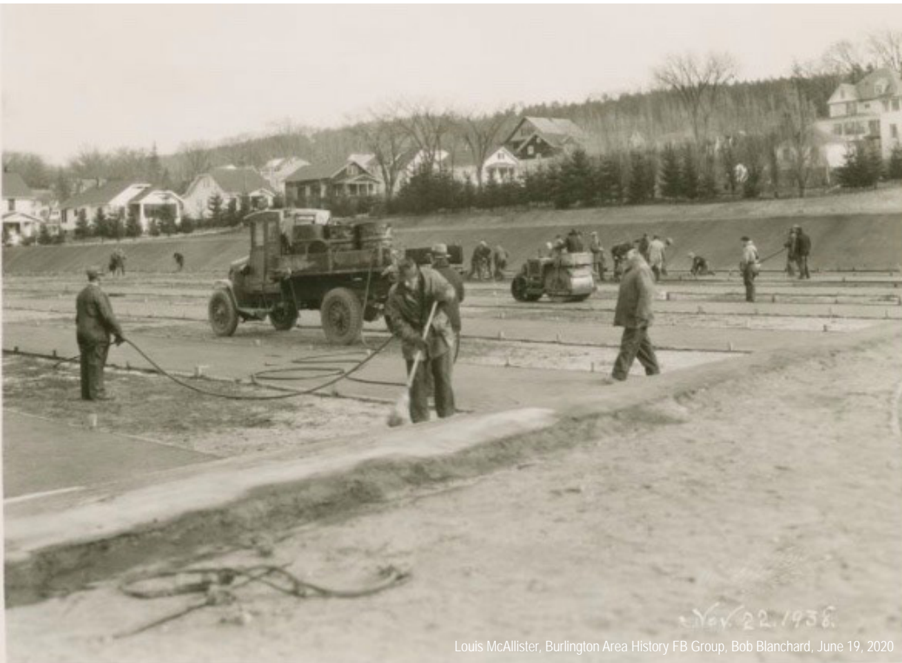
1938 - Tennis Court Installation
