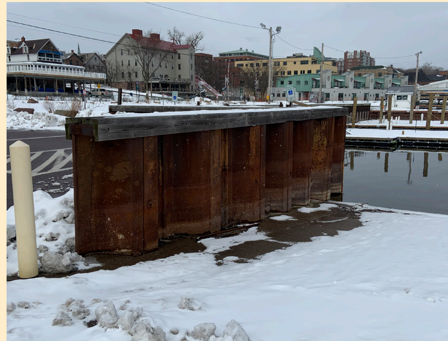
STEEL SHEET PILE
